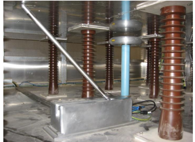
Figure 5: The automatic earthing arm and voltage divider under the high voltage platform.
