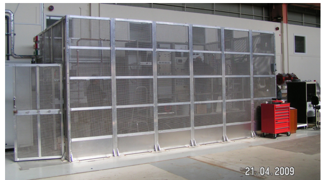
Figure 2: High voltage cage completed.
